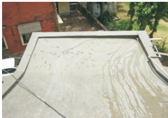
After application of Flexi-Crete
