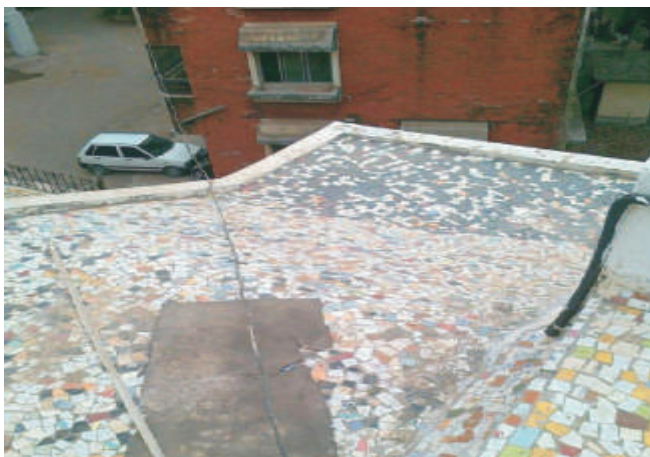
Before application of Flexi-Crete
